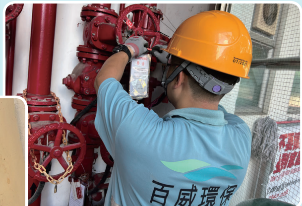
Description: Worker was performing fire service system checking
