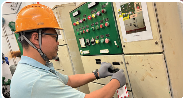
Description: Worker was performing fire service system checking
